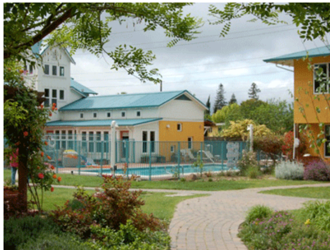
View of Pool and Common House from First Street
